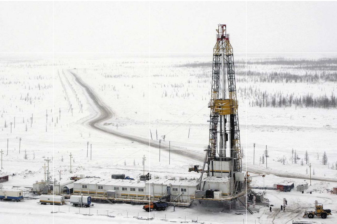
Well pad No. 4 at the Vankor field
