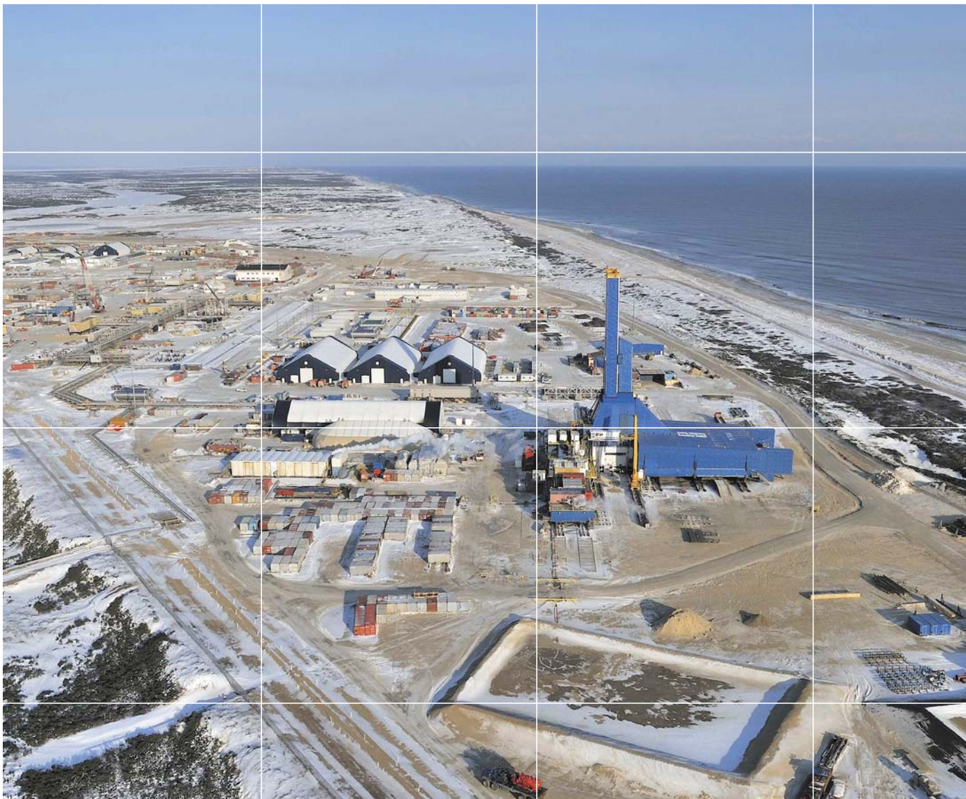
Production drilling at the Odoptu field as part of the Sakhalin-1 project
