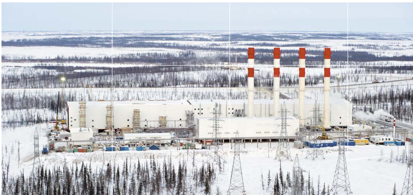
Gas-turbine power station at Vankor
