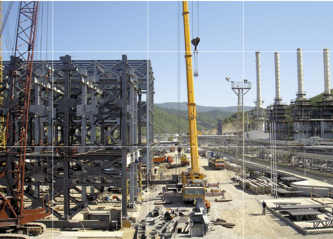
Construction of a crude distillation unit at the Tuapse refinery
